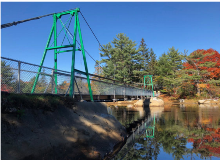
SABLE RIVER FOOTBRIDGE
